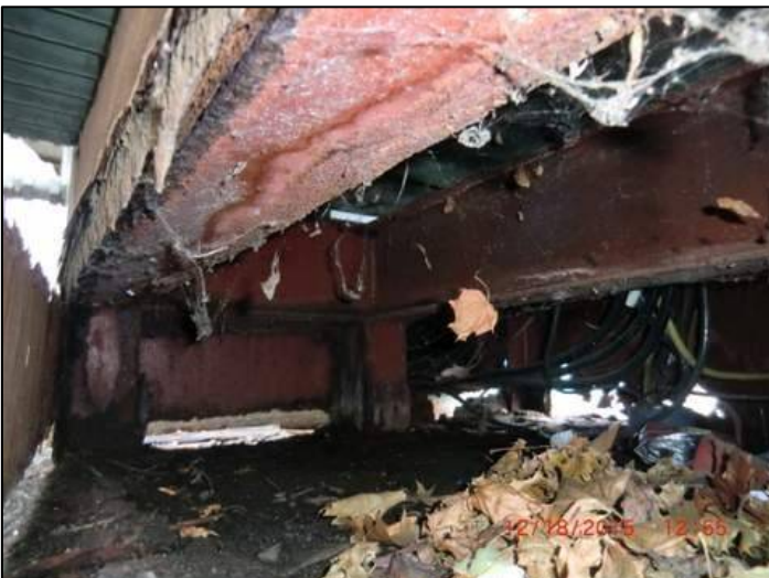
⑨ The view to the south through the rusted out opening on the rear northeast corner. There appears to be at least one set, perhaps two, of large 3 phase conductors running down from the transformer bus area, through the short connecting raceway to the terminal box. It's not clear whether LU's primary voltage supply line to the transformer arrives through an underground conduit from under the transformer in this area or in the base of the terminal box.
