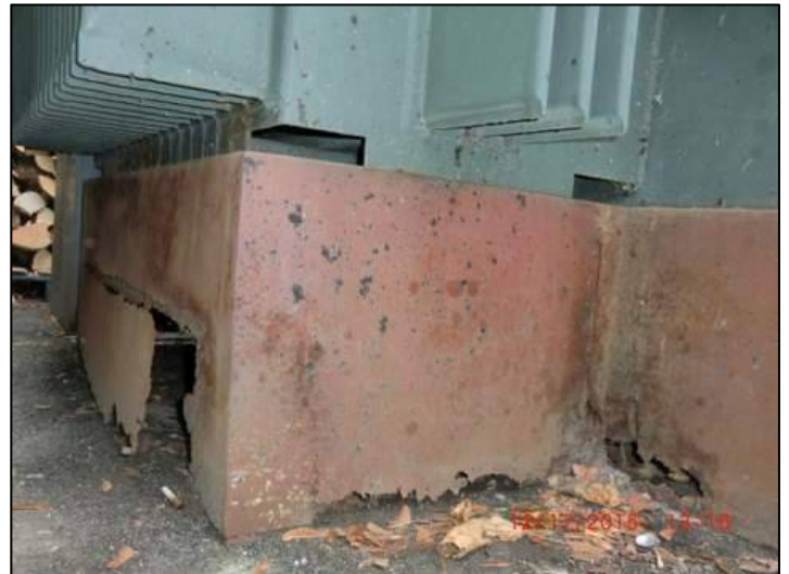
⑧ LU's transformer base from the northeast rear corner. Cigarette butts and dry leaves under the transformer could be a dangerous combination. The two photos below were taken through the flapping hole seen on the lower left. The steel structural tubes holding up the steel I-beams are on the outside rear corners
