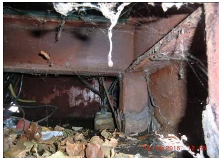
⑩ The view under the base from just outside through the rear hole. Note the spalling rust on the square tube structural support. The conduit in the front of the transformer (center back of picture) appears to host grounding conductors, probably to a ground rod or grounding cable. Except for the ground conductors there do not appear to be any splices in this area under the transformer.
